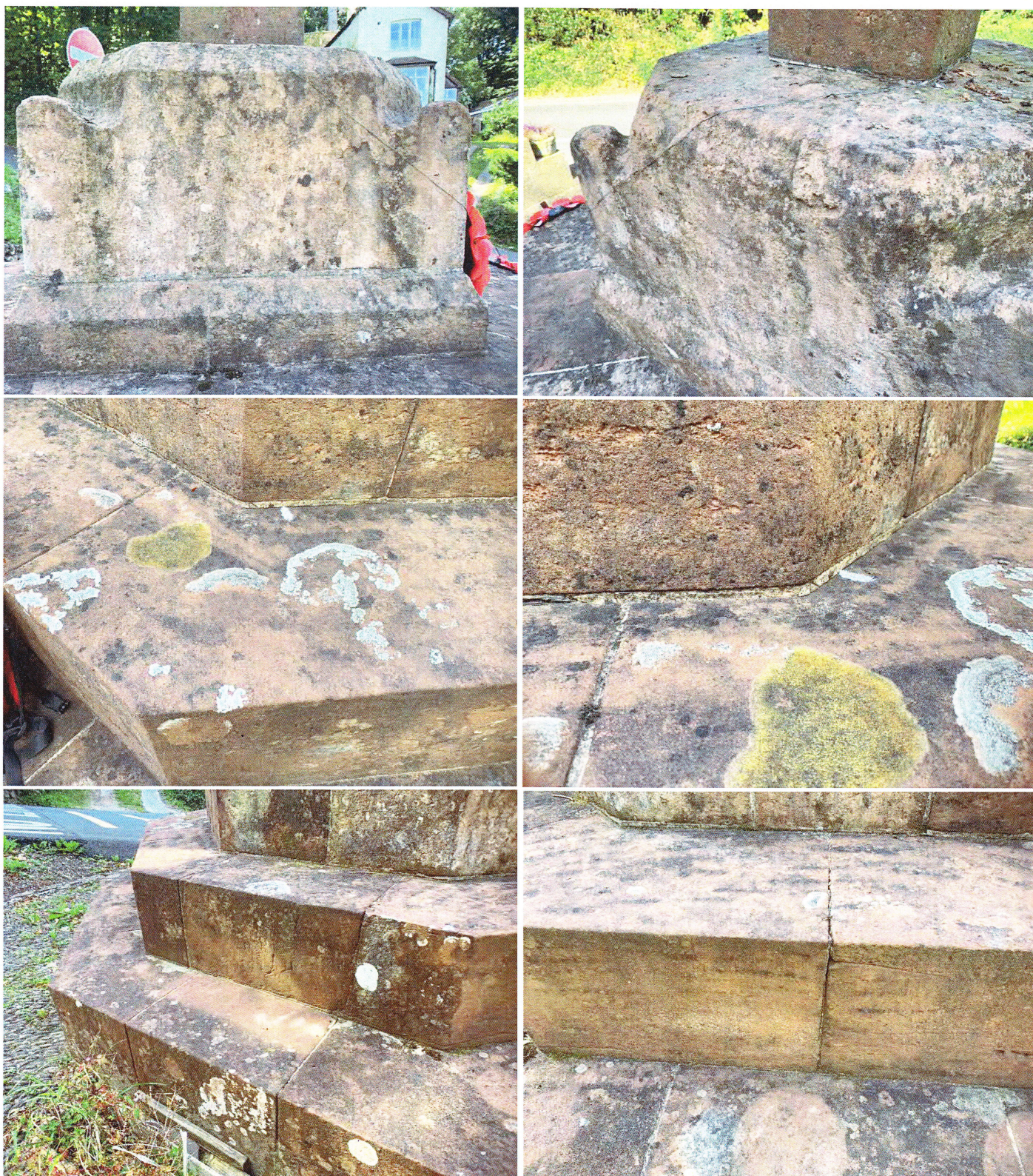
General areas showing the surface condition of the main memorial - clear indications of vegetational and biological growths (lichens, algae etc) as well as pollutants and general air-borne debris.
